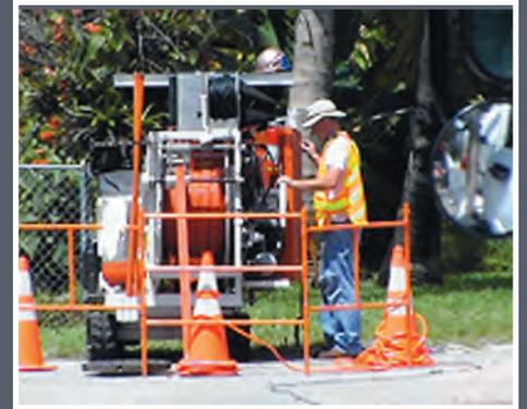
T-Liner® can be installed in main pipe diameters ranging from 6 to 30-inches and lateral pipe diameters ranging from 3 to 12-inches while negotiating multiple bends and pipe diameter transitions. Best of all, the main and lateral portions of a T-Liner® are resin saturated, inserted, and cured all at the same time producing a truly homogenous structural lining that incorporates gasket sealing technology and provides a verifiable non-leaking connection.
