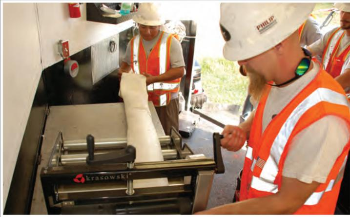
LMK's T-LINER® is constructed from a one-piece engineered textile producing a structural Main/Lateral lining tube. The lining tube is positioned inside of the patented translucent inversion bladder. This translucent bladder allows the installer and inspector to visually verify the liner is thoroughly saturated with a thermo-set resin during the vacuum impregnation process, therefore ensuring there are no dry spots.
