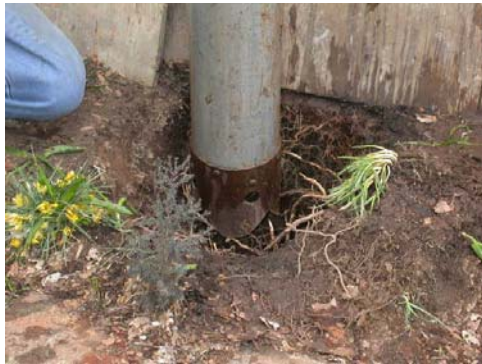
Figure A Error! No text of specified style in document.-1 Hydro excavating of the pit
