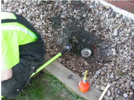
Figure A Error! No text of specified style in document.-3 VAC-A-TEE® Cleanout installed in the pit
